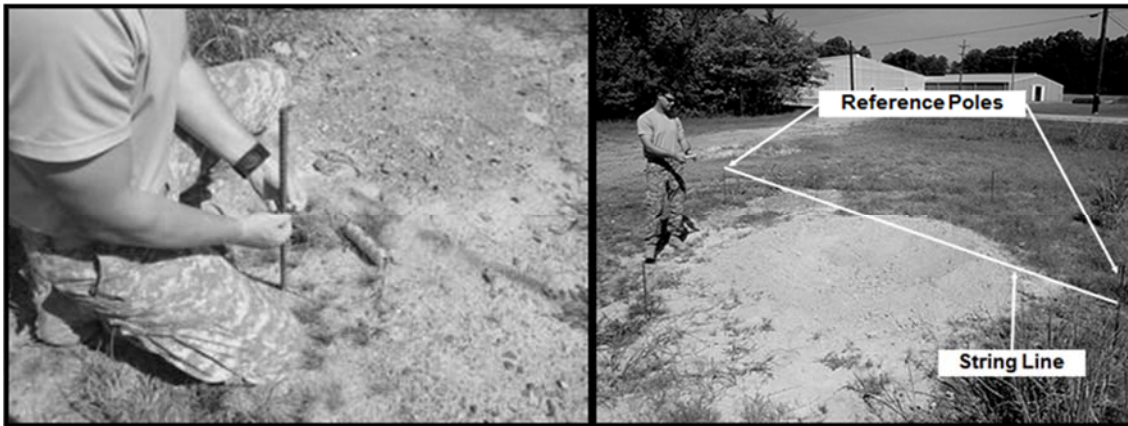
Figure G-9. Step 2. Establish reference data points
